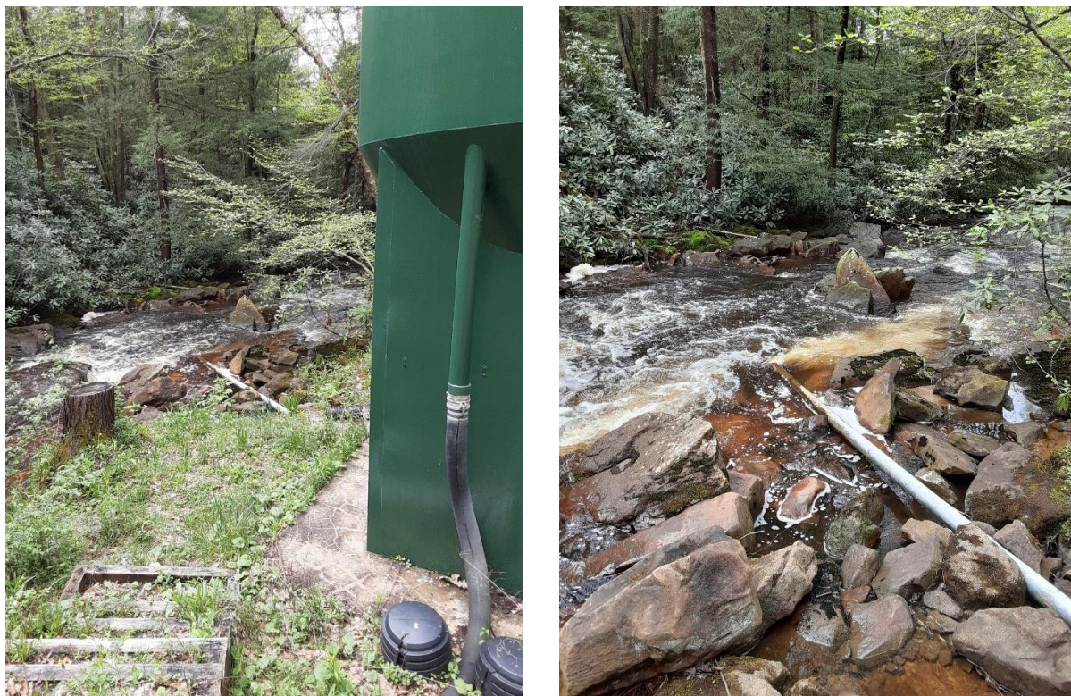
Figure 3 – Images of limestone doser located on Cherry Creek, upstream of its confluence with Deep Creek Lake.
